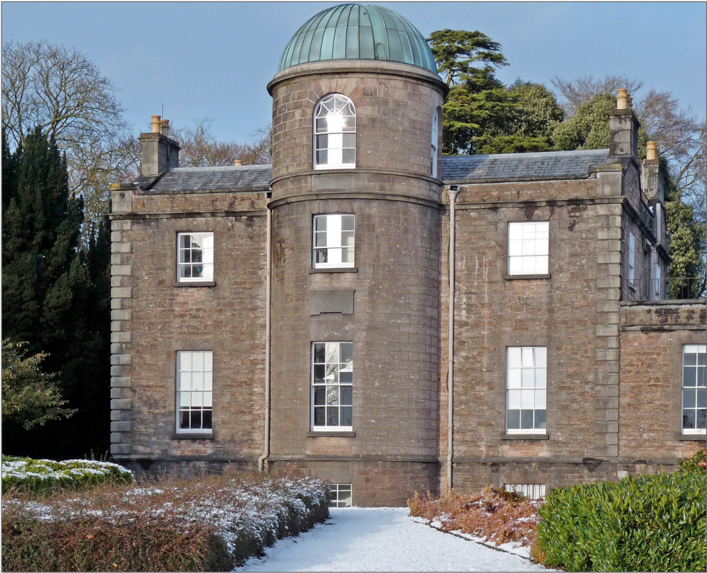
Figure 3. South elevation of Armagh Observatory showing the Troughton dome and location of the first OSBM to the right of the lower ground floor window of the dome and 2.7 feet below ground level. Image taken on 2009 December 21. Image credit Mark Bailey.
