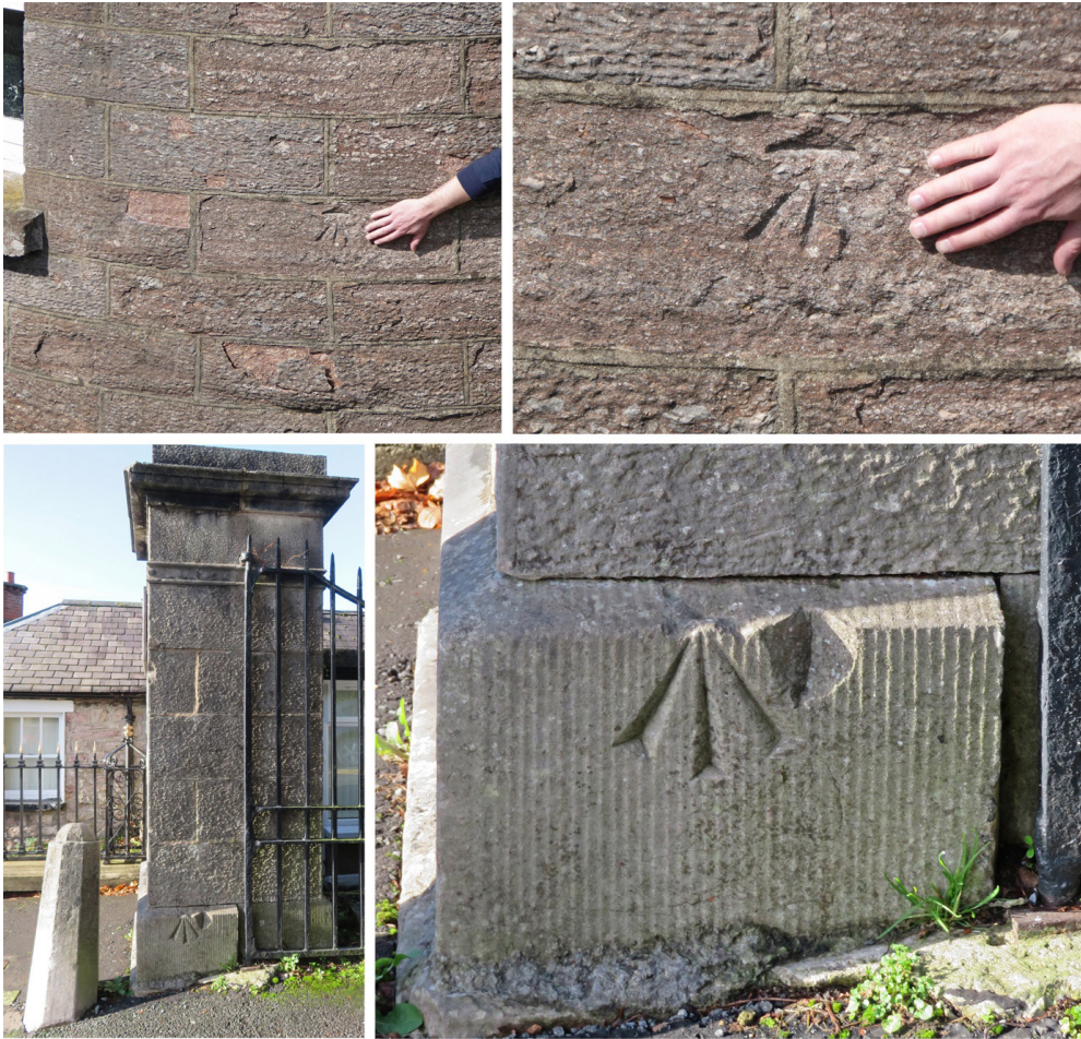
Figure 4. Top left: Location of OSBM #1 to the right of the basement window and on the south-east face of the Observatory's Troughton telescope dome. Top right: Detail of this OSBM, image taken on 2016 April 21. Lower left: OSBM #2 at the foot of the western gate post at the entrance to the Observatory grounds near the Gate Lodge. Lower right: Detail of OSBM #2. Image credit: Mark Bailey.
