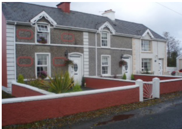
Figure 4: These extant two-storey, terraced labourers' cottages situated in Stranorlar RD, Co. Donegal were based on the standard Model Plan G. (Photo: Frances Crampsie, Oct 2007).
