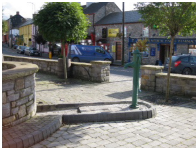
Figure 3: An early twentieth century water pump restored to its former glory in the centre of Virginia, Co. Cavan. Pumps similar to this appeared across the country in the early twentieth century as rural district councils sought to provide a clean water supply for local populations. (Photo: Arlene Crampsie, Oct 2008).
