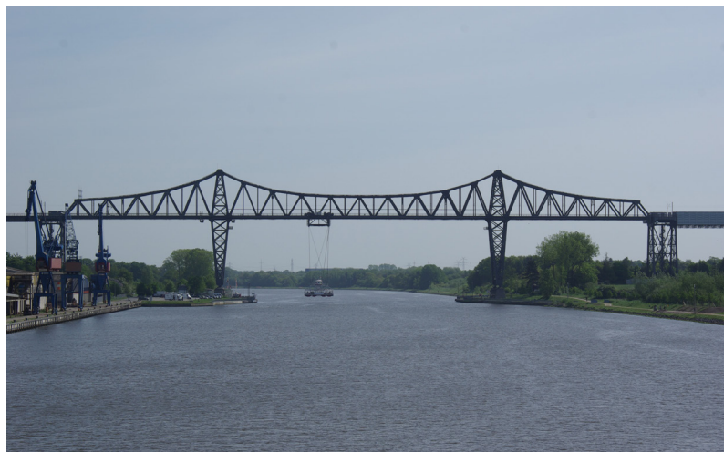
Figure 7. The Eisenbahnhochbrücke Rendsburg – a surviving example of a transporter bridge. The gondola now can carry four cars. Wikimedia Commons
